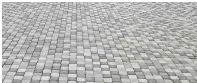
Key Vehicle / Pedestrian Intersections Small unit concrete sett paving, silver grey Example Product: Charcon Countryside Classic
