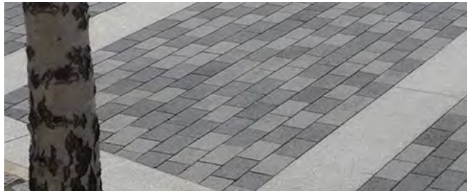
Key Public Spaces Textured concrete paving blocks, mix of greys Example Product: Charcon Andover Textured
